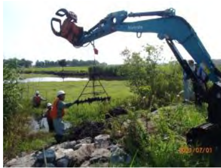
Figure 4. A backhoe “swing-yarder” originally used for forestry work, with a specially made rake.
