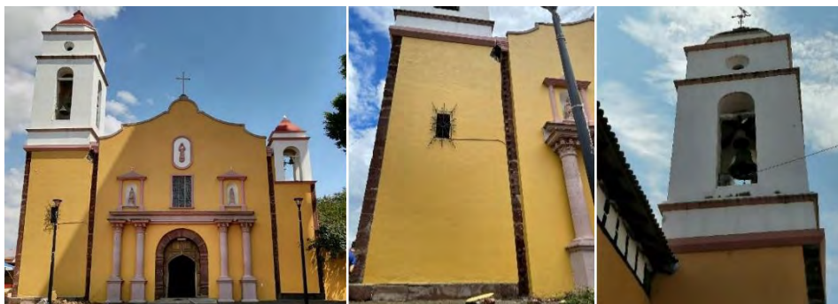
a) Fachada principal
